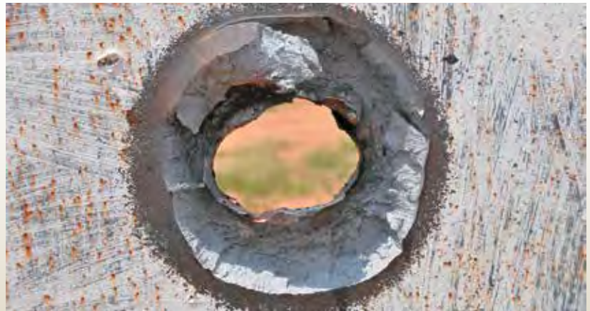
Typical damage or penetration caused due to an improvised explosive device projectile on an unprotected target.
