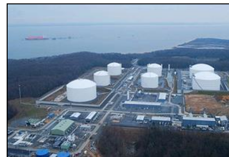
Dominion Cove Point LNG terminal with a capacity of 0.4 bcm storage (LNG); 18.6 bcm/a regasification
