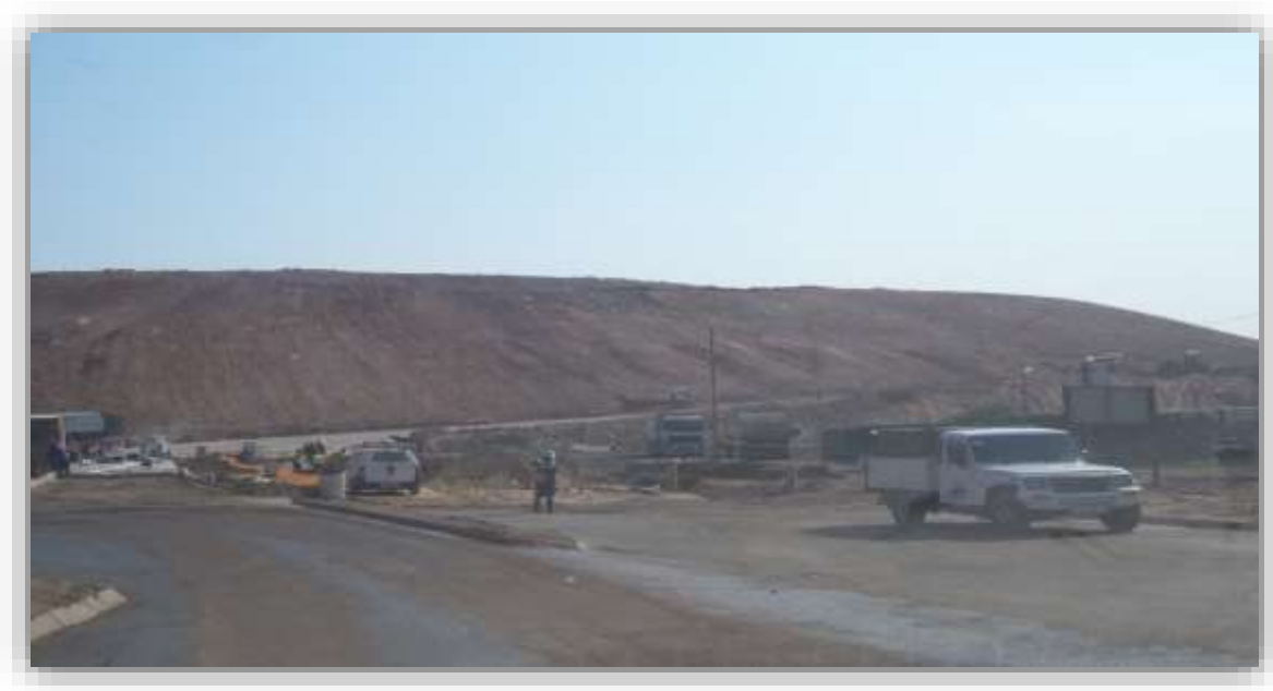
Figure 5: Weighbridge still being constructed at Robinson Deep landfill site.
