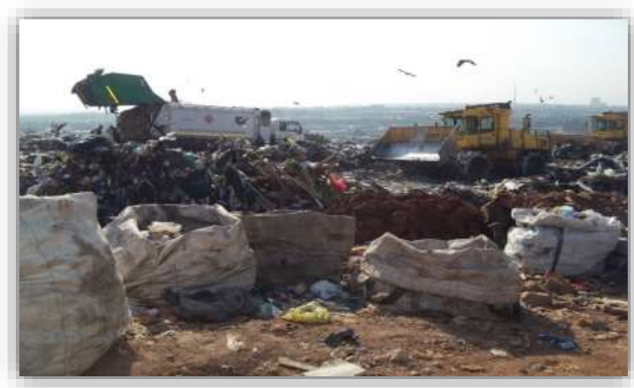
Figure 8: Pikitup truck off-loading the waste at the tip of the phase, reclaimers collecting and separating waste and compactor truck compacting waste.
