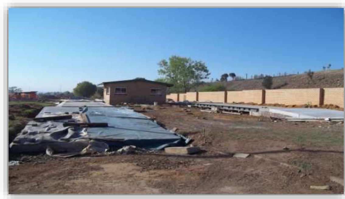
Figure 4: Marie Louis Weight Bridge under construction
