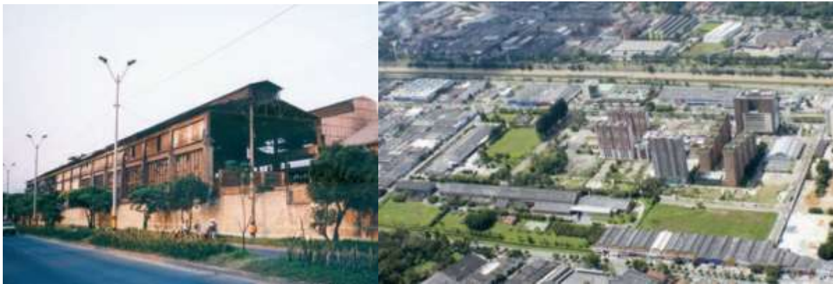
Image (Left): One of the former steel mills on the site in 2006 Image (Right): Aerial view of the Simesa project under construction in 2011.
