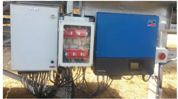
Figure 4: Typical Thin Film Configuration for the Inverter at ERIC
