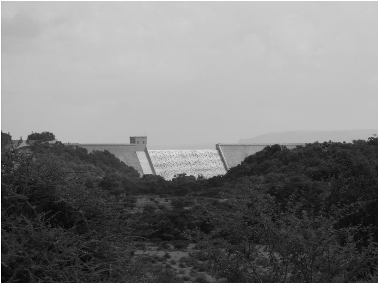
Figure 1: The De Hoop Dam (©Richard Meissner)
