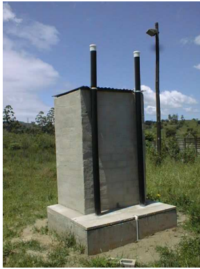
Photograph 1. Typical double vault urine diversion toilet in the Durban area
