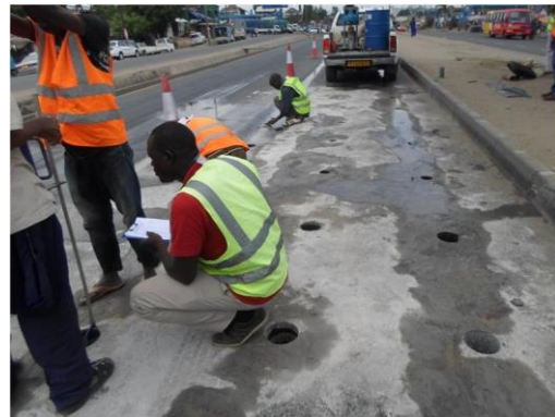
(b) DCP tests at core positions
