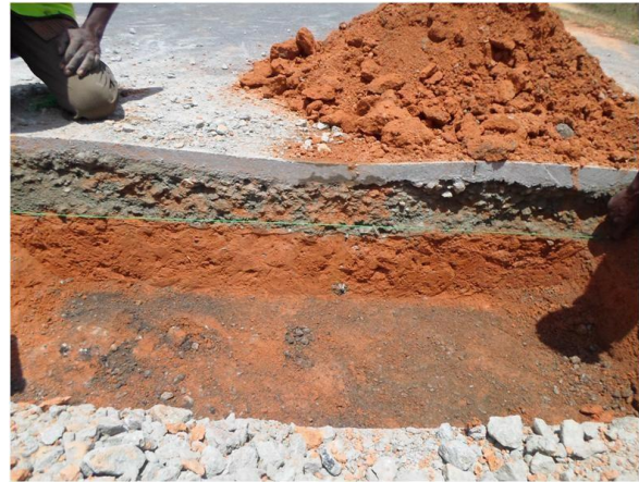
(b) Test pit at Iringa-Mafinga road section
