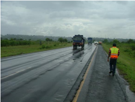
(a) Severe rutting on Mlandizi-Chalinze road section
