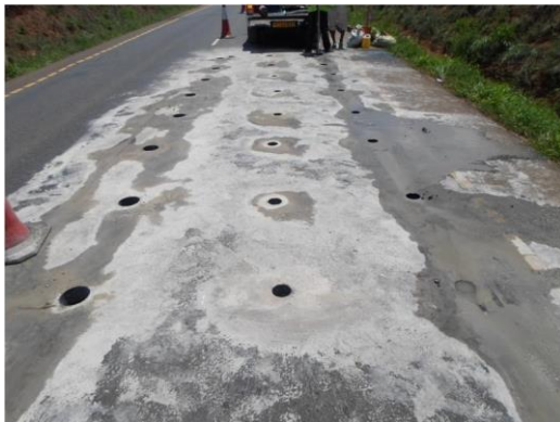
(a) Core position and holes for a road section
