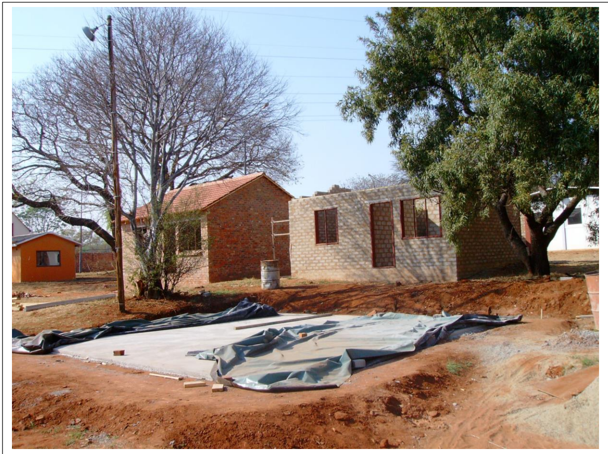
Figure 3: Ultra-thin concrete raft slab
