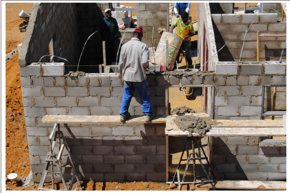
Figure 4: CSIR designed house, Kleinmond
