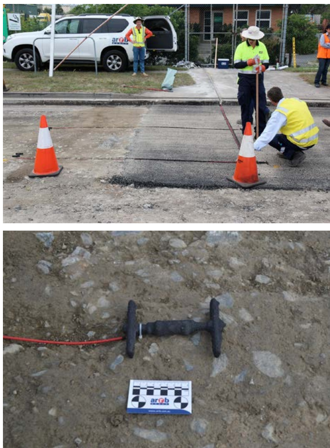
Fig. 6. Strain gauges being installed in the pavement
