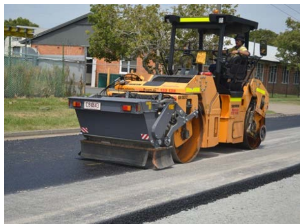
Fig. 5. Gritting of the EME surface
