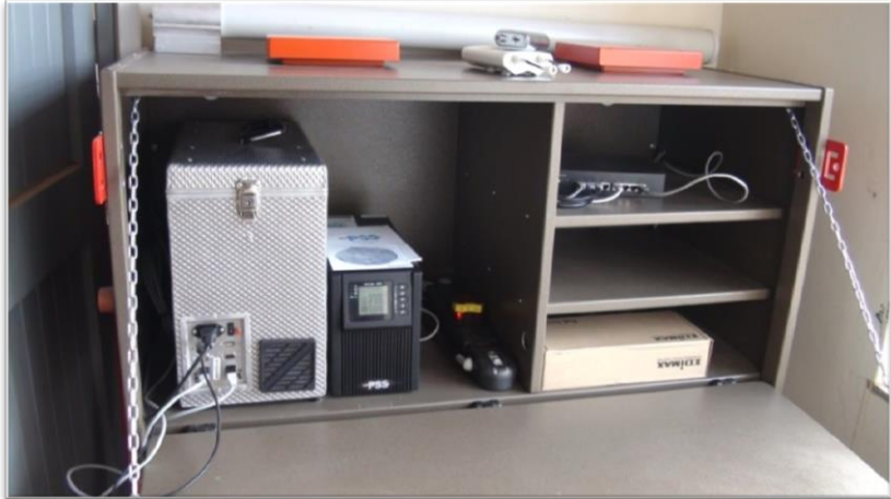
Photo 4-2: The silver box is where the server was placed in a secure, folding container which had to be placed in a secure and ventilated area in the school.
