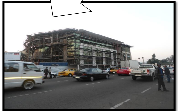
Figure 10: Tourism Hub under construction August 2013 (Google Earth: 2013)
