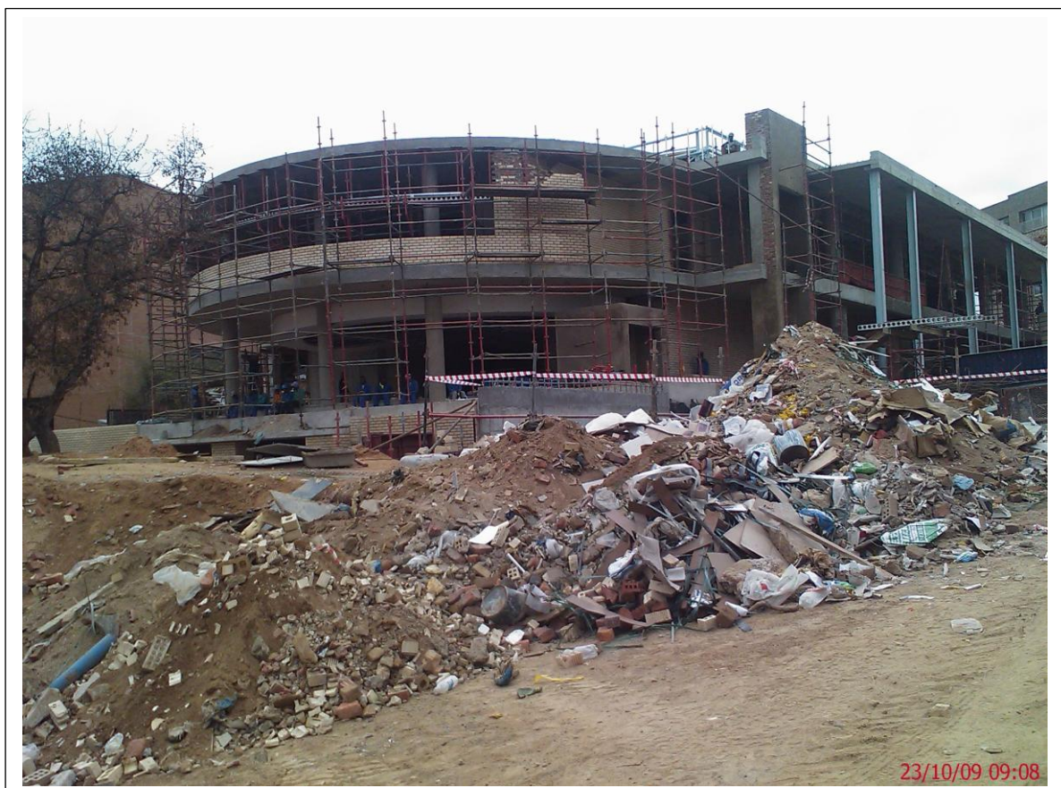
Figure 1: Example of construction waste on a typical construction site
