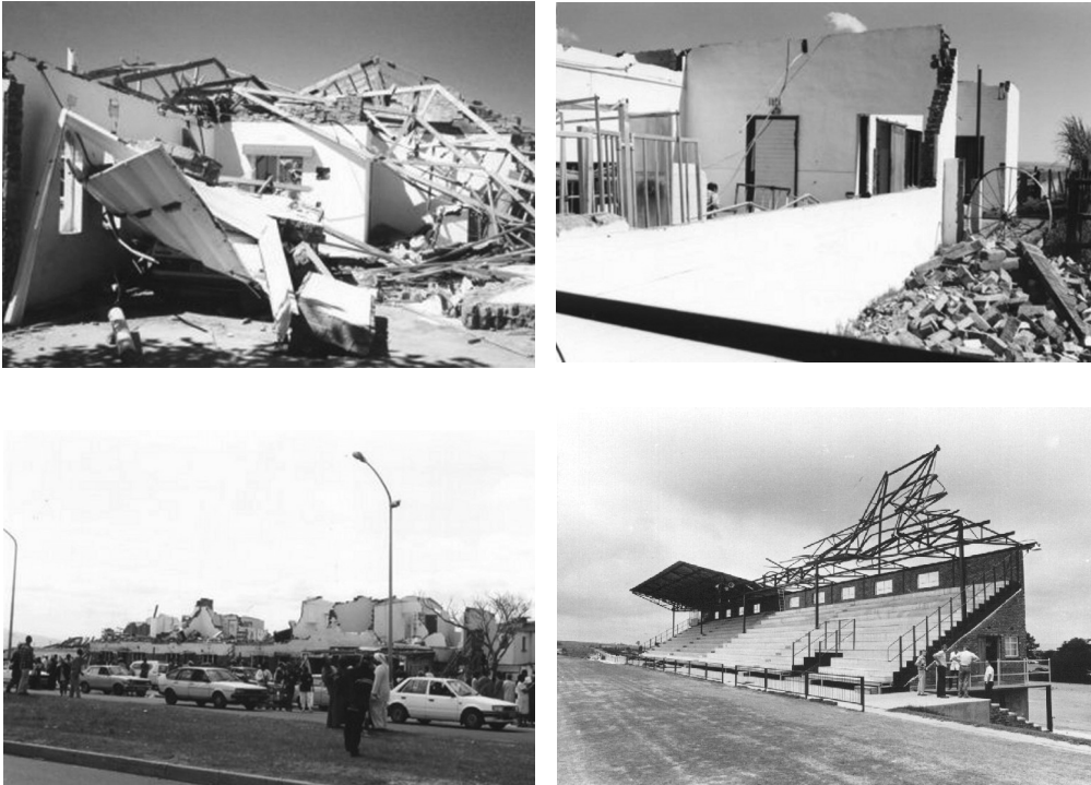
Fig. 20. Examples of serious damage in South Africa.
