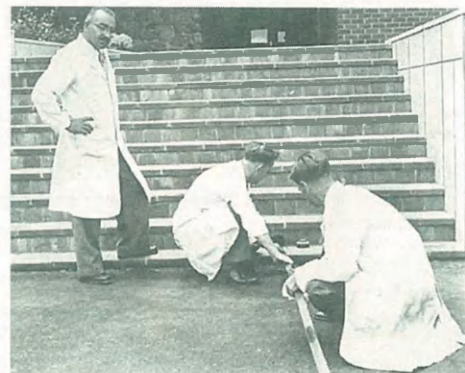
NML staff 'walking' the 50 m steel length bar from the CSIR workshops and passing it into the tape tunnel through a secret hole in the steps up to the new NPRL building (Jan 1960)
