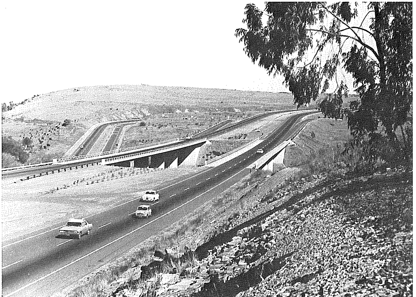
A recently constructed dual-carriage highway.
