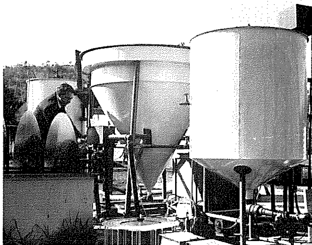
A pilot plant for the anaerobic digestion of raw sewage.
