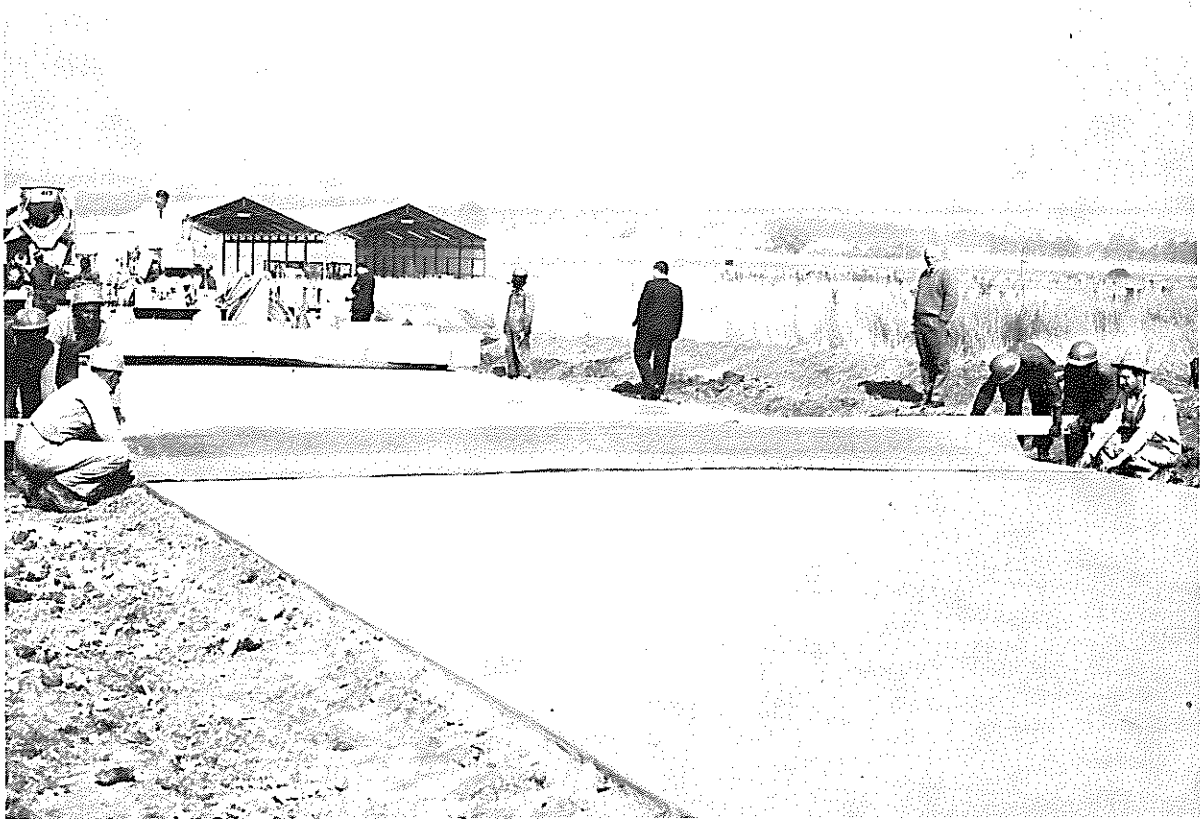
A section of an experimental concrete road being laid at the NIRR's test site in Pretoria
