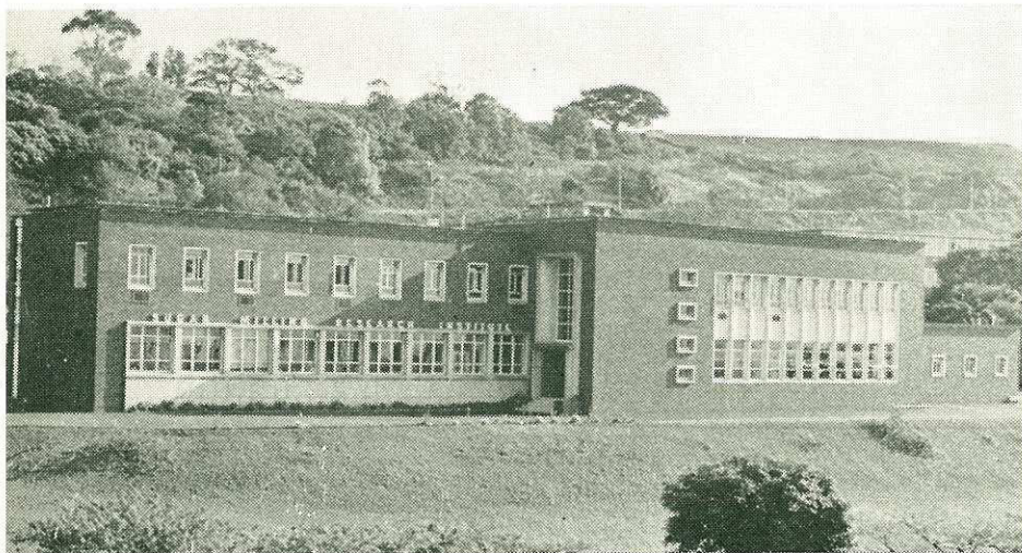
The Sugar Milling Research Institute building in Durban.
