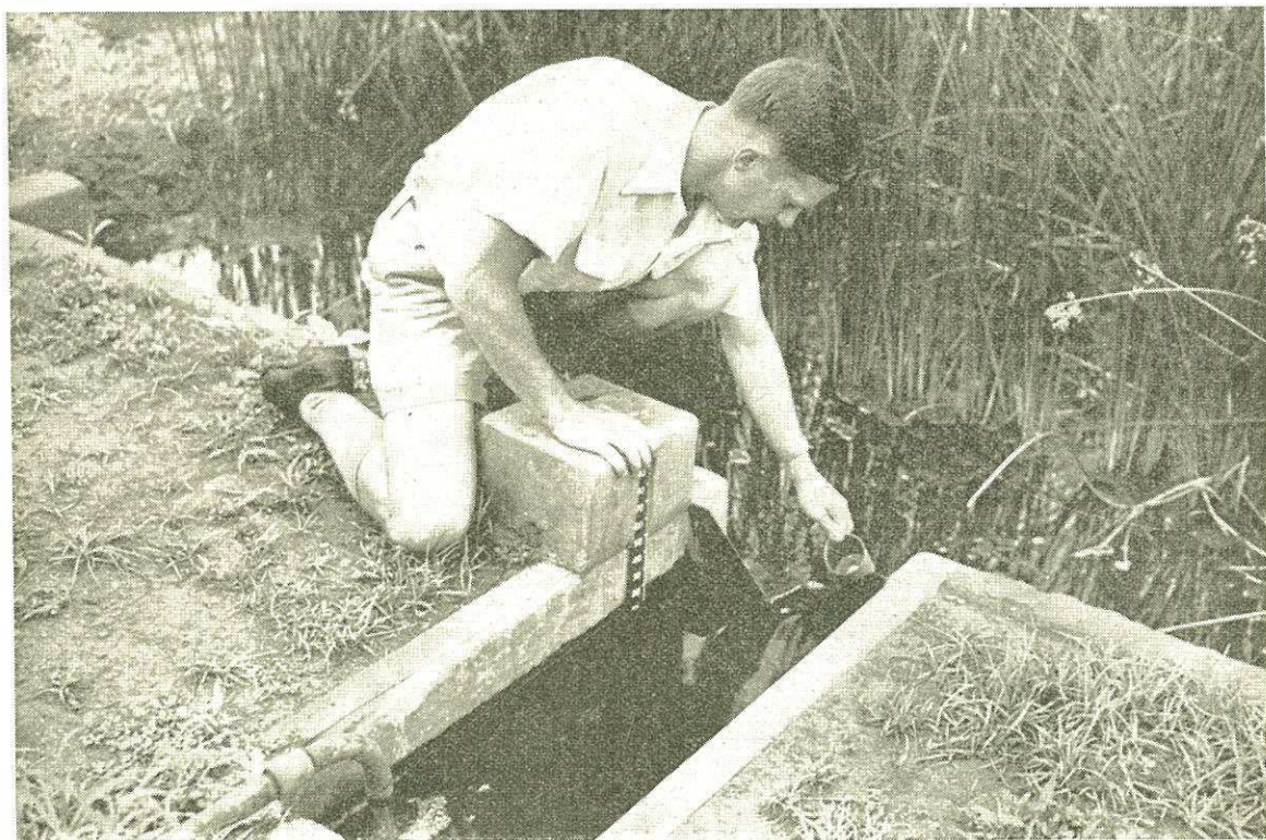
Taking a sample of sewage works effluent as it flows into an artificial vlei, where it undergoes further purification prior to re-use.
