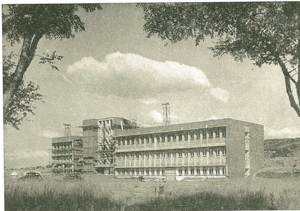
The new nuclear physics building under construction at the new C.S.I.R. site seven miles east of Pretoria. The ventilators for the cyclotron hall, which is 30 feet below surface, can be seen in the left foreground.
