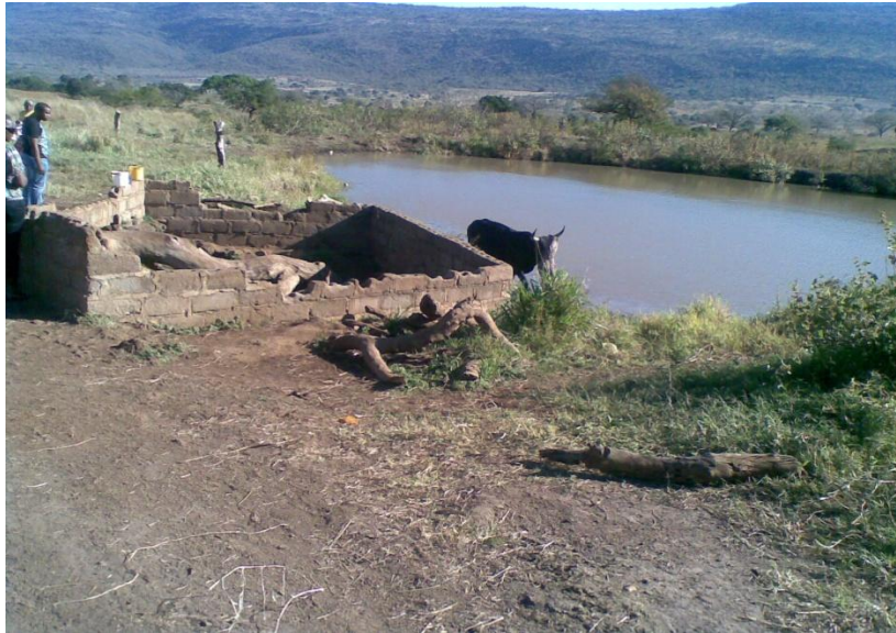
Figure 18: A photo of a fountain which is used for drinking, cooking and cleaning, a wall has been constructed to protect from livestock
