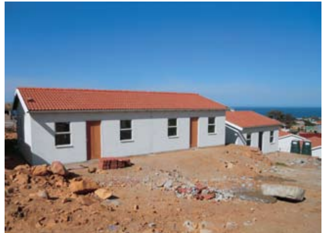
Houses under construction in Kleinmond, using many CSIR-developed features.
