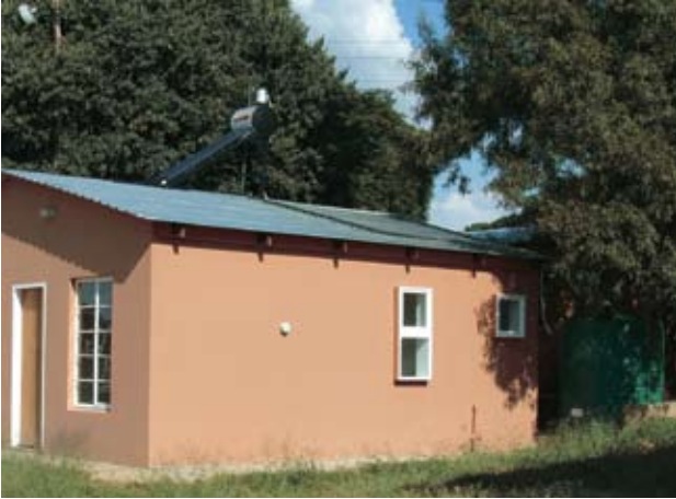
The CSIR's demonstration unit for improved government-subsidised low-income housing.
