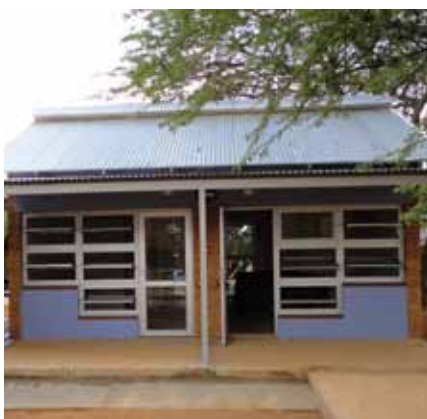
A typical MDR-TB block at Modimolle Hospital.
