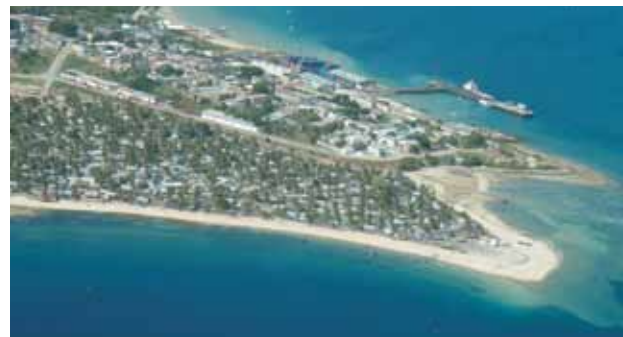
Pictured is the highly vulnerable area at the north-western tip of the city of Pemba in Mozambique, where the village of Paquite is regularly threatened by sea inundation.
