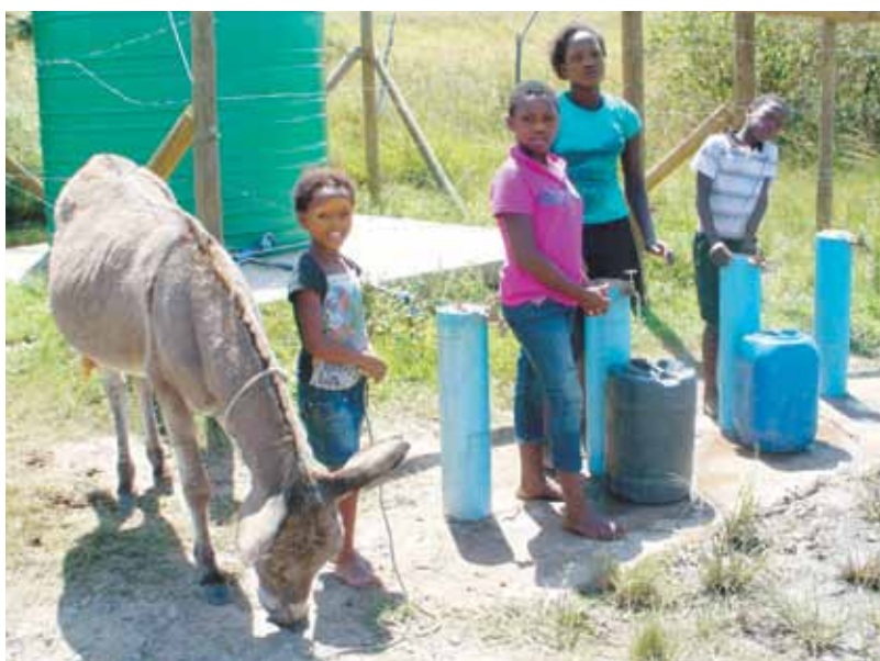
Children from the nearby community collecting safe, sustainable drinking water from taps. The water is pumped from the communal water station to a small storage tank, from where gravity carries the water in pipes all the way to taps in the village.
