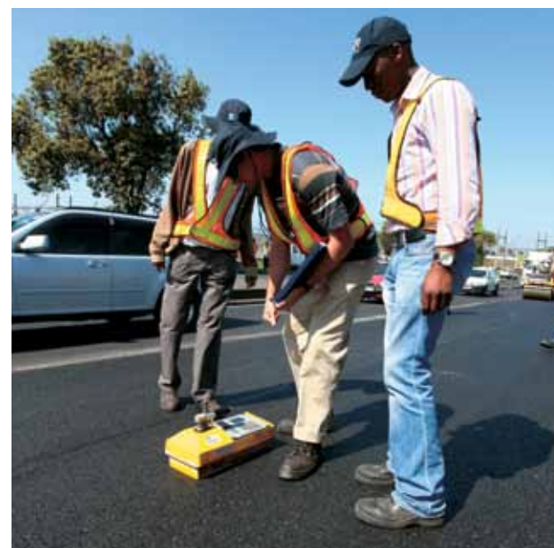
A density gauge is used to measure the density of the compacted high-modulus asphalt layer; optimal density ensures optimal performance.
