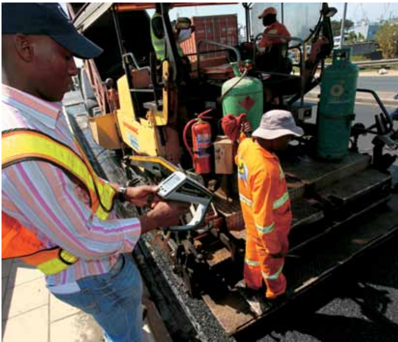
Tso Nkgapele of the CSIR with an infrared thermal imager to obtain a two-dimensional image of the surface temperatures of the high-modulus asphalt. Temperature control is important to attain the correct degree of compaction.
