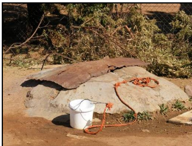
Figure 3.4: Typical South African protected borehole with small bucket used as a scoop.
