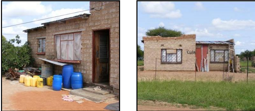
Figure 3.3: Typical brick houses with corrugated iron roofs common in the area
