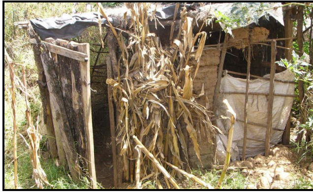
Figure 4.5: A Kenyan rural communal toilet.
