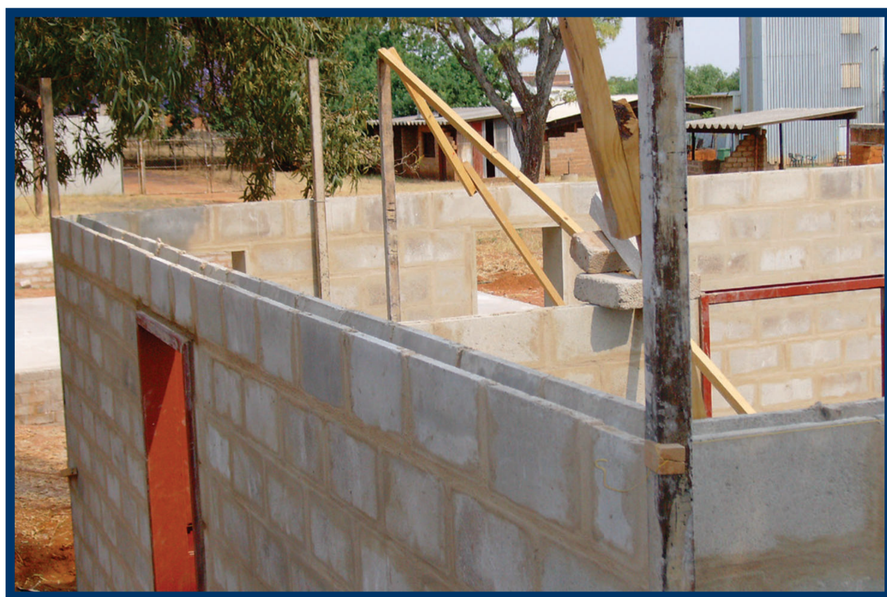
Figure 2: Construction of brick building
