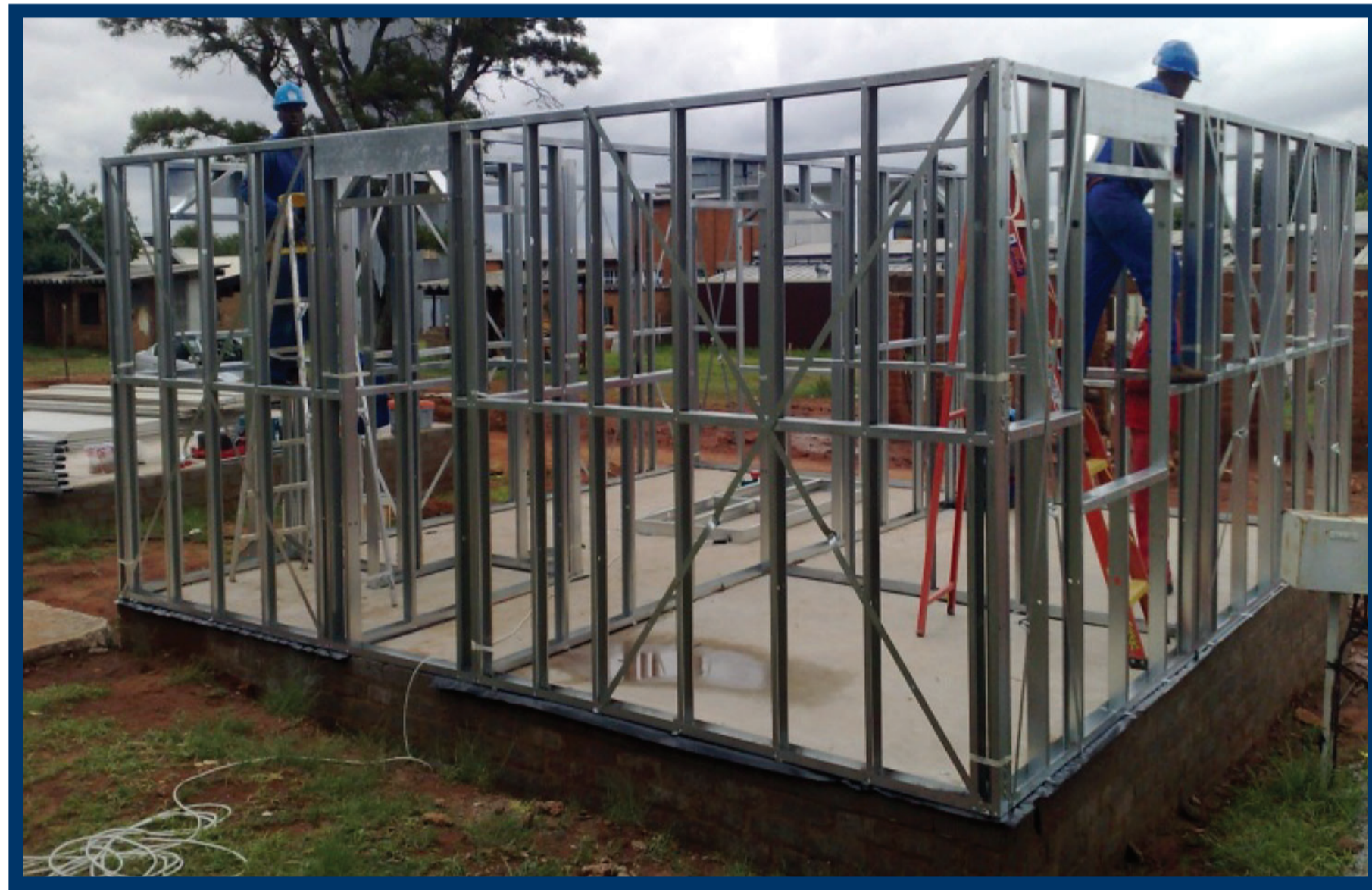
Figure 1: Construction of a Light Steel Frame (LSF) building
