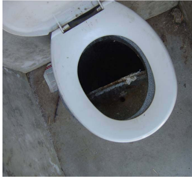
Figure 20: Outdoor UDD toilet for the maintenance team of the SPHC (Source: CSIR, 2011).
