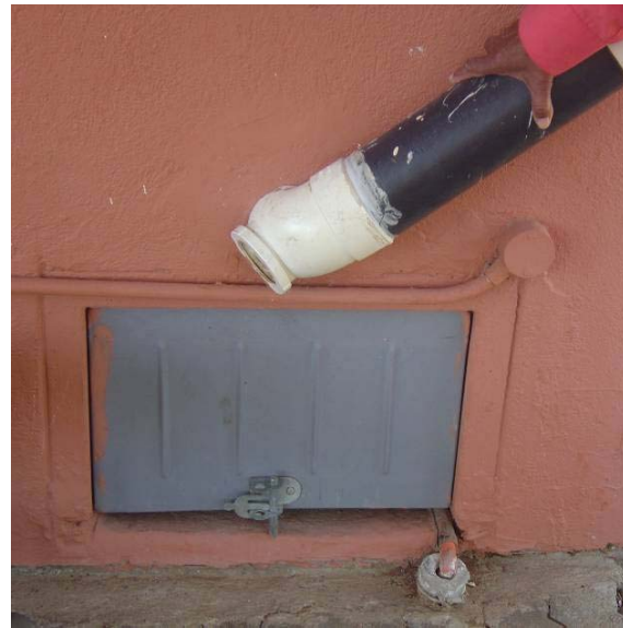
Figure 18: Door to access a faecal vault from outside the housing unit (Source: CSIR, 2011).
