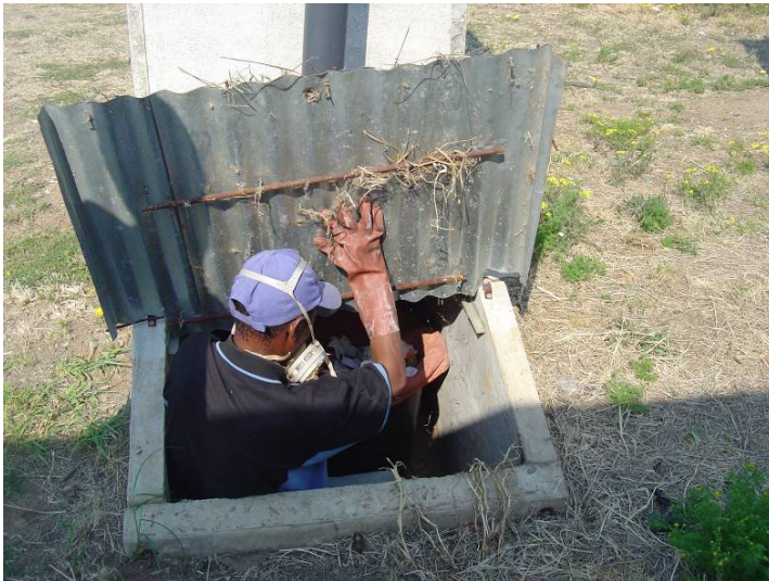
Figure 9: Maintenance team member empties a faecal drum of the outdoor toilet at SPHC (Source: CSIR, 2011).
