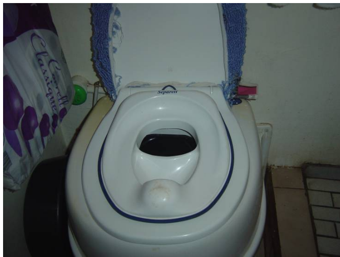
Figure 3: Example of UDD toilet with a kiddie seat in Hull Street (Source: CSIR, 2011).
