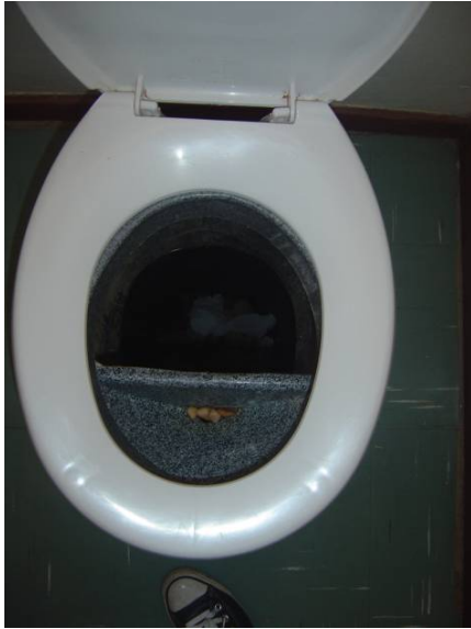
Figure 19: Indoor UDD toilet for office staff at the SPHC (Source: CSIR, 2011).
