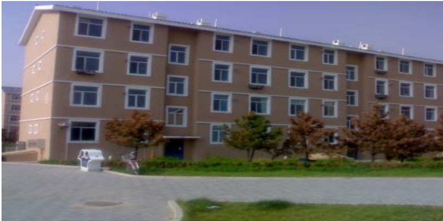
Figure 4: MDMH development with UDD toilets, China-Sweden Erdos Eco-town Project (EETP), China (Source: McConville and Rosemarin, 2011).
