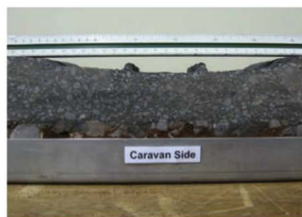
Figure 5b: This road sample displays rutting or plastic deformation in asphalt surfacing. Heavy Vehicle Simulator (HVS) tire loading of 20kN, and inflation pressure of 800kPa (with typical "n-shape" vertical stress distribution), resulting in typical "n-shape" plastic deformation in a thin asphalt surfacing layer – only one HVS tire traffic lane is shown here 23
