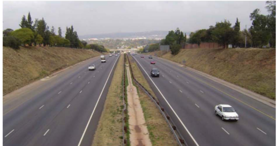
Figure 1: An aerial photograph of a high-quality thin surfaced divided freeway located near Pretoria, South Africa
