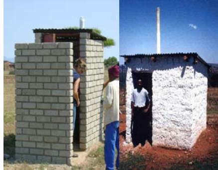
Figure 3 Superstructures constructed from cement bricks, wattle and/or adobe (CSIR and DWAF, 2007)
