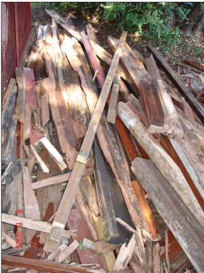
Structural damage to untreated wood
