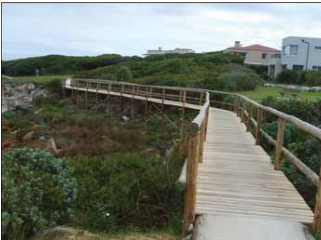
The town of Onrus now boasts a new bridge thanks to the efforts of Jip Margadant of Wood Solutions
