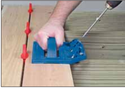
Place the Kreg screw into the deck jig collet and drive the screw in
