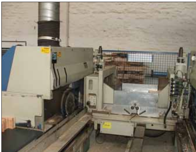
The squaring and finger-joint cutter unit on the Grecon finger-joint line
