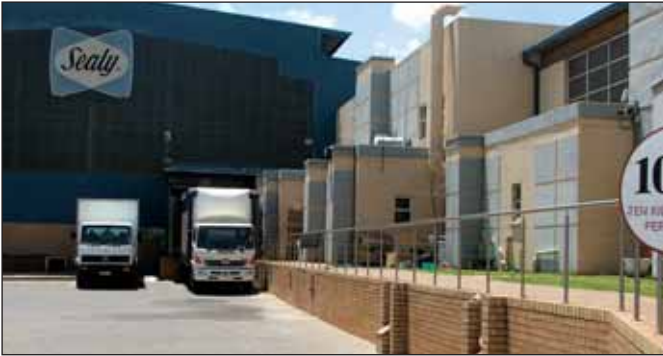
The Bravo Sleep Products Group's manufacturing headquarters located in Industria west of the Johannesburg city bowl
