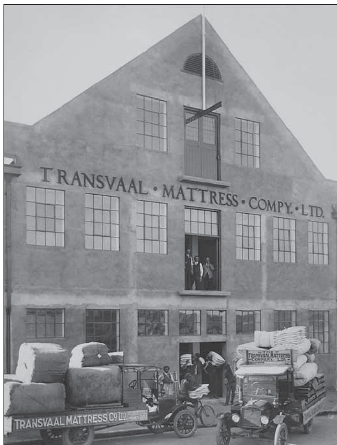
The old Transvaal Mattress Company building
