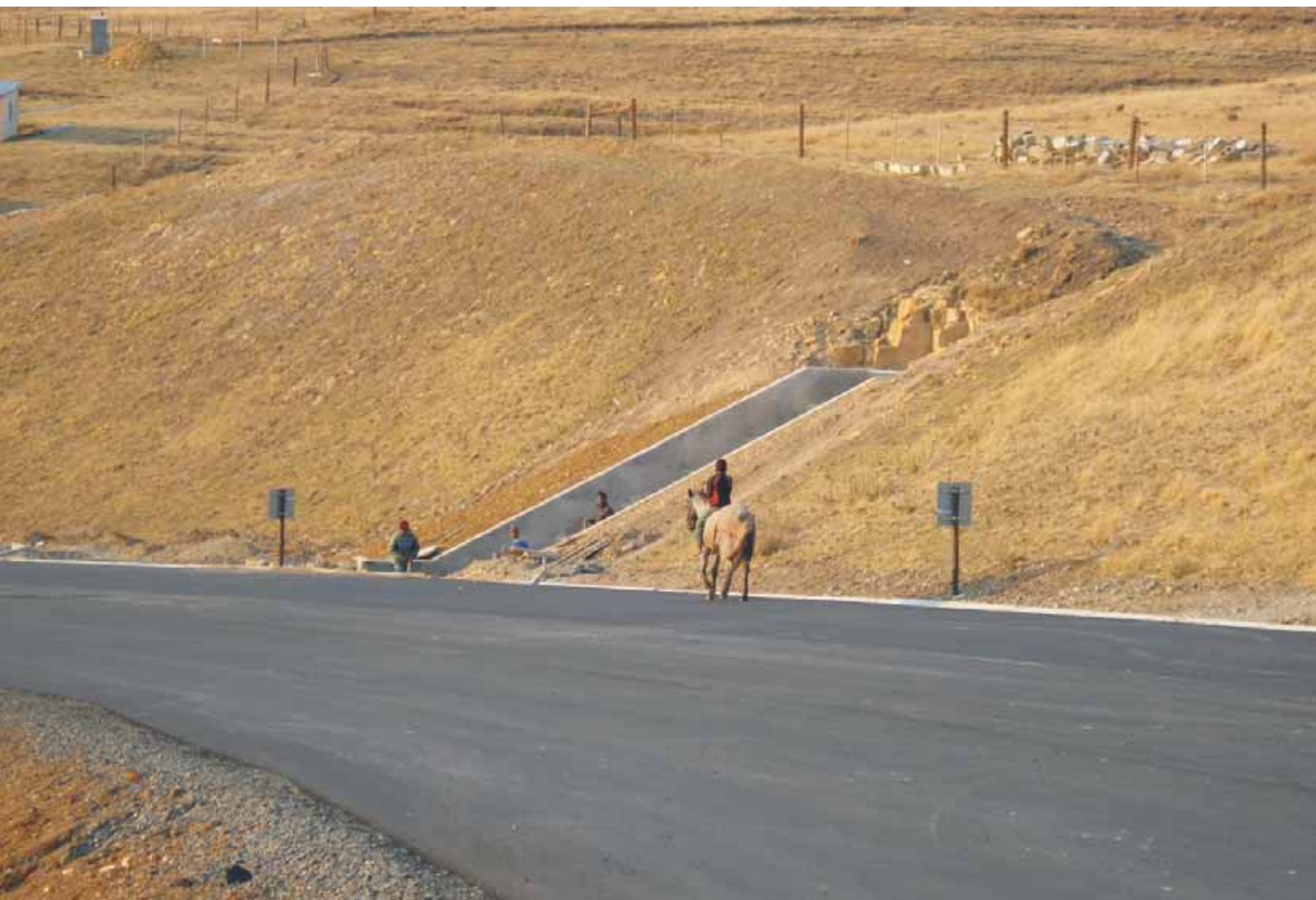
Contrast between modern technology and rural access needs
