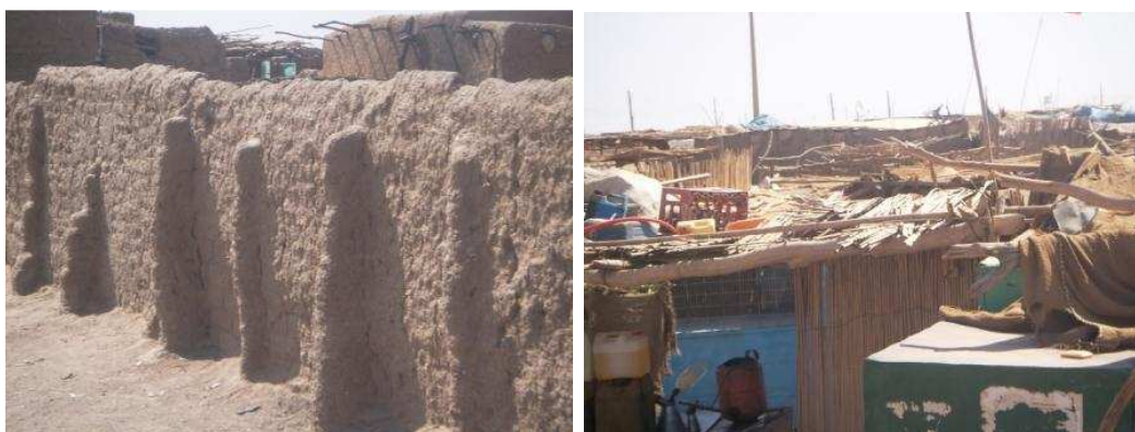
IMAGES 1 AND 2 TYPICAL "ISHASH" OR SHANTY TOWNS ON THE PERIPHERIES OF KHARTOUM – CONSTRUCTION USING POLES, MUD, FABRICS, TINS OR ANY FOUND MATERIALS
