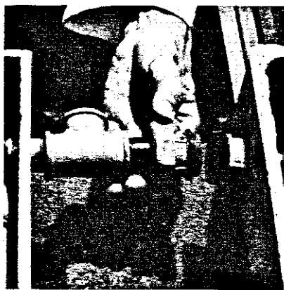
13. Remove tile and fit interconnecting pipes.
