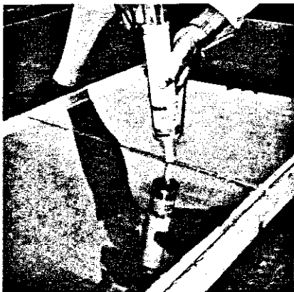
27. Position adjacent sheets of glass within 1-2 mm of each other and fill this gap with silicone sealer.
