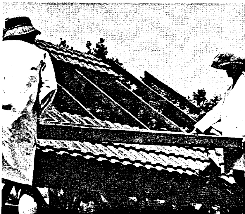
5. Place asbestos cement tray on roof. If more than one panel is required, assemble pipe fittings to establish position of other trays (see page 38 and step 13).
