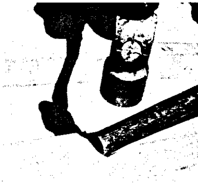
17. Fixing on an IBR or corrugated steel roof can be done by cutting a slot with a cold chisel and using a steel pipe to form a depression.
