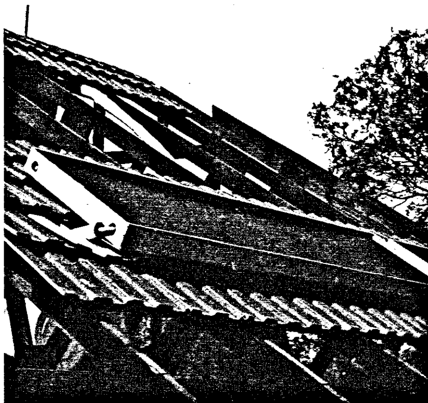
31. The completed job for a sloping roof.
