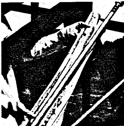
28. Cover flow and return lines with glass-fibre or polystyrene insulation. Any exposed insulation should be covered with steel muffs.
