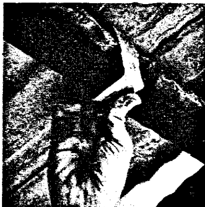
9. Tray can also be secured with steel strapping. This can be slid between overlapping tiles and saves drilling through tiles.
