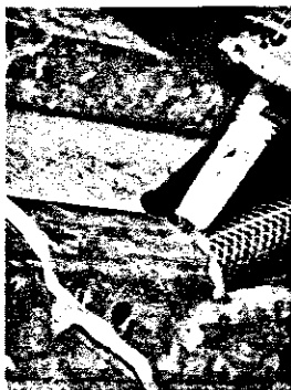
18. Pass hosing or steel pipe through hole and seal with silicone sealer.
