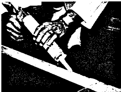
25. Spread silicone sealer along top edge of asbestos cement tray.
