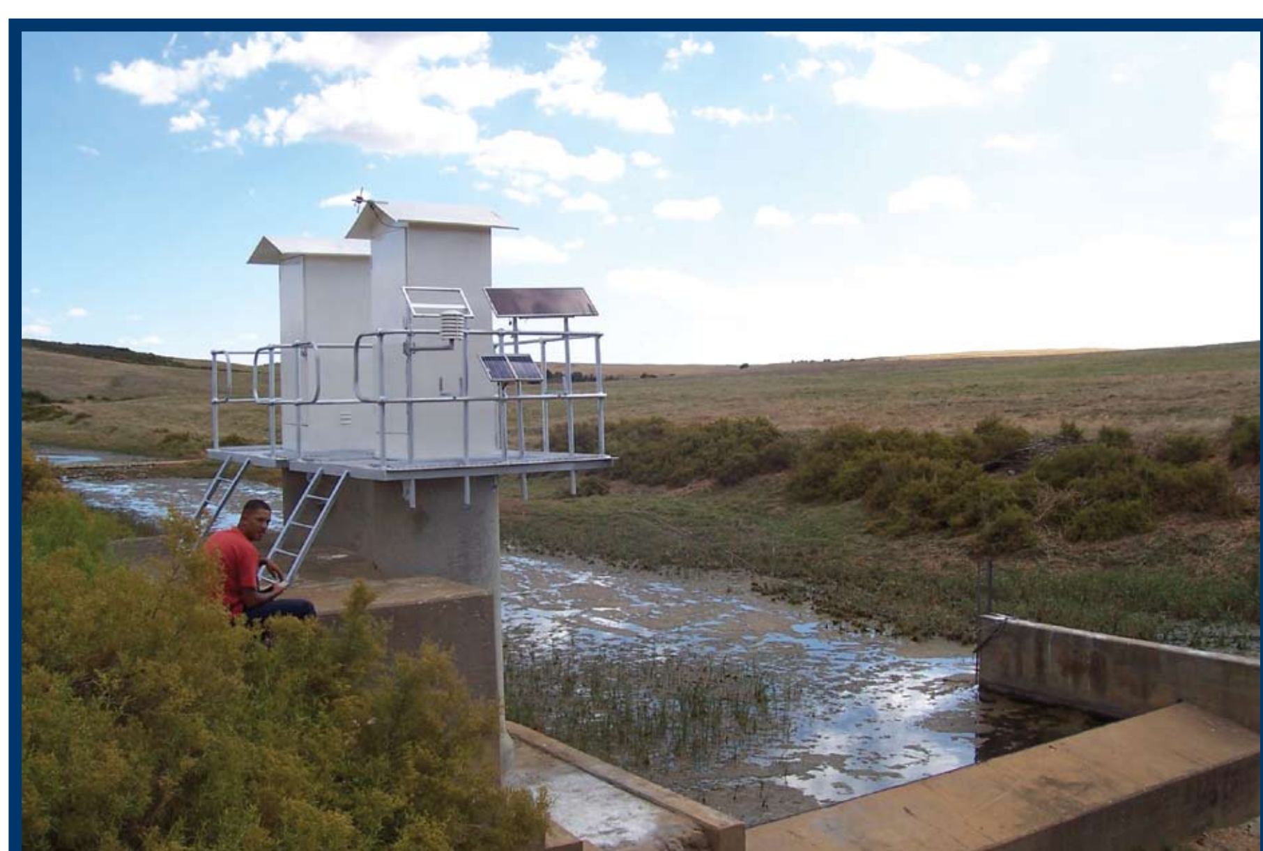
Figure 2: The flow monitoring station at the outlet of the Sandspruit catchment
