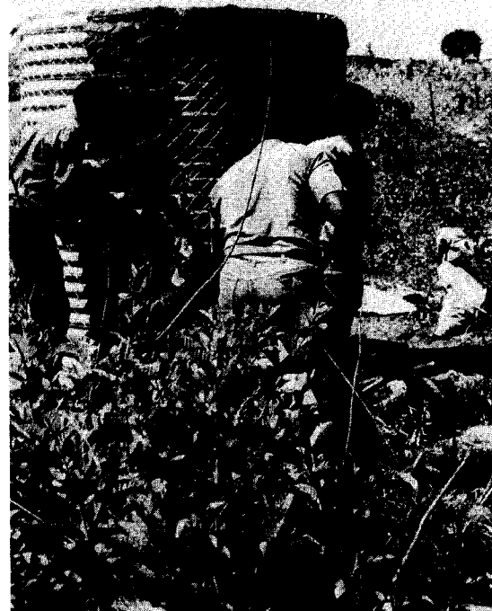
Fig. 13b Building a ferro-cement tank
