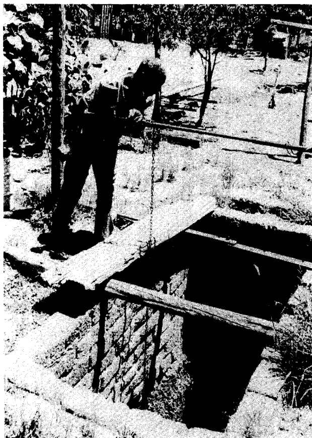
Fig. 11. This well is contaminated by buckets being lowered into it.
