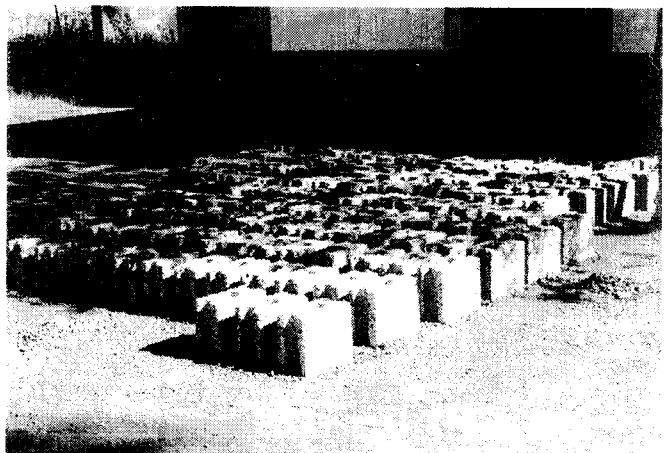
Block production for a tank
