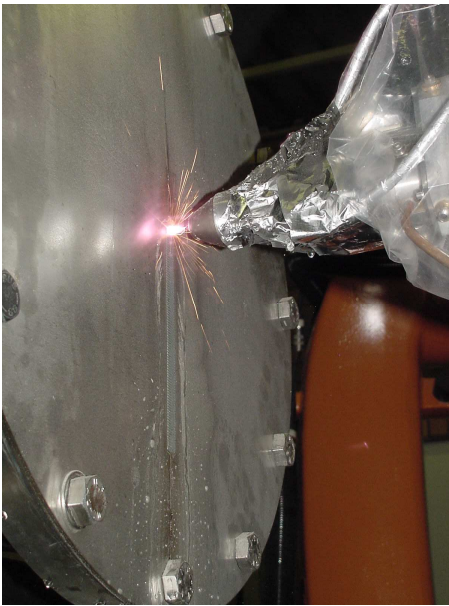
Fig. 4: Crack sealing of 4.5 mm plate @ 2 bar pressure
