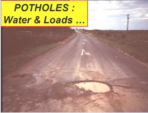
Sub-grade Failures...
