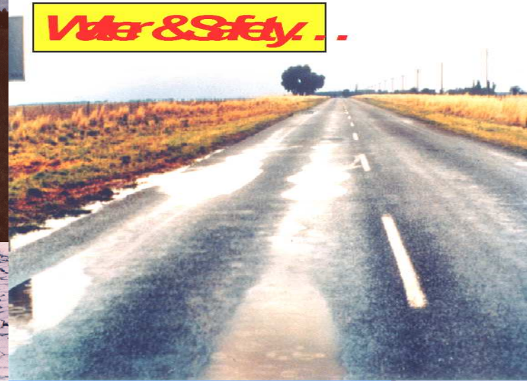
SURFACE DISINTEGRATION
