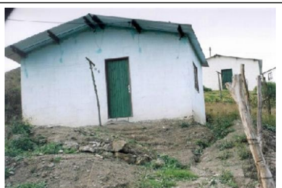
Subsidy housing, Mooiriver – one year after construction
