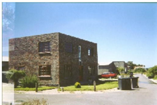
House built through the People’s Housing Process, Victoria Mxenge, Cape Town Source: S. Liebermann, CSIR
