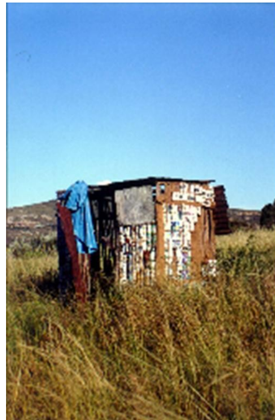
Rural sanitation: wattle, can and daub pit latrine, Naledi Village Source: C. du Plessis, CSIR
