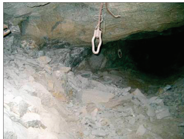
Figure 10—Pillar 14 and the fractured rock in the ASG after the burst
