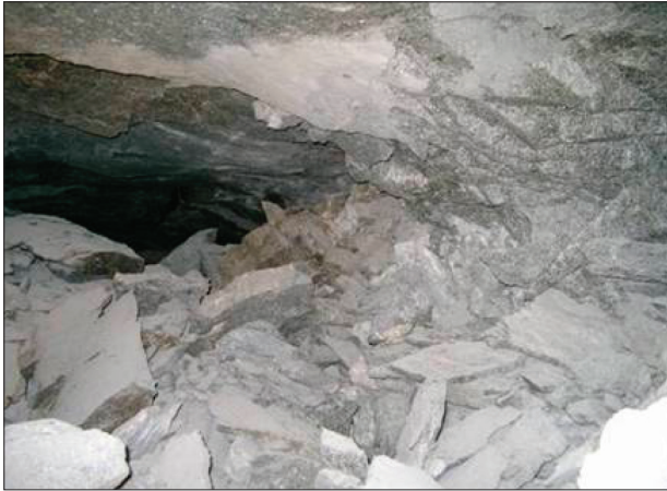
Figure 12—Up-dip side of Pillar 16
