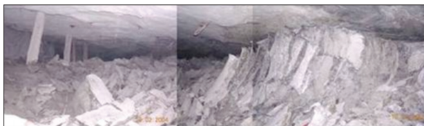
Figure 2—Panoramic view showing the up-dip end of a burst pillar. Note the gully is full of rock fragments from the pillar burst
