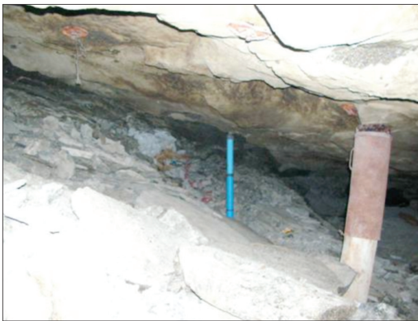
Figure 13—Down-dip side of the instrumented pillar. View away from face
