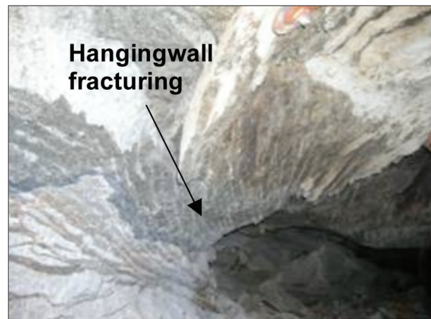
Figure 16—Up-dip side of the instrumented pillar. View towards face
