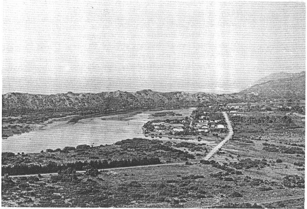
FIG. 15: The central section of the estuary with the Swartvlei peninsula in the middle of the picture. Note the steepness of the vegetated dunes and their proximity to the estuary channel. A low, inadequate causeway in the road crossing the Perdespruit where it joins the Swartvlei estuary can be seen in the centre right of the photograph. (IFWS: 83-03-08).
