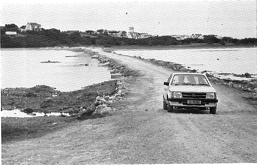
FIG. 11: The weir/causeway across the Seekoei Estuary with Paradise Beach Township in the background. The impact of the causeway is clearly evident. (Photo: ECRU: 83-05-16).
