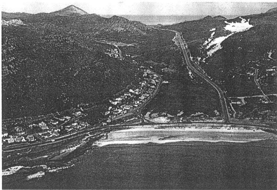
PLATE II: The Elsie's River mouth, showing to what extent the roads and railway line dominate the lower part of the estuary. Open water can be seen in the Vlei and the remnants of the original bare dune belt are visible on the top right-hand corner of the photograph. The Glencairn township is on the left with the new subdivision of Glencairn Heights on the right (ECRU 79-10-23).
