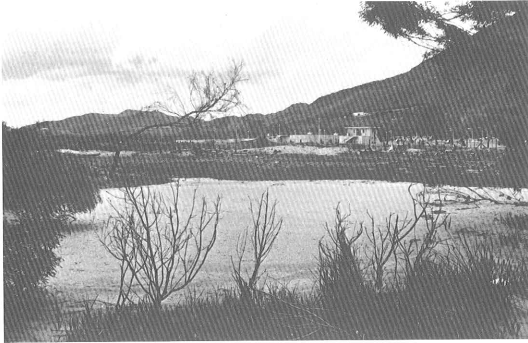
FIG. 8: The Wildevoëlvlei sewage treatment works.
