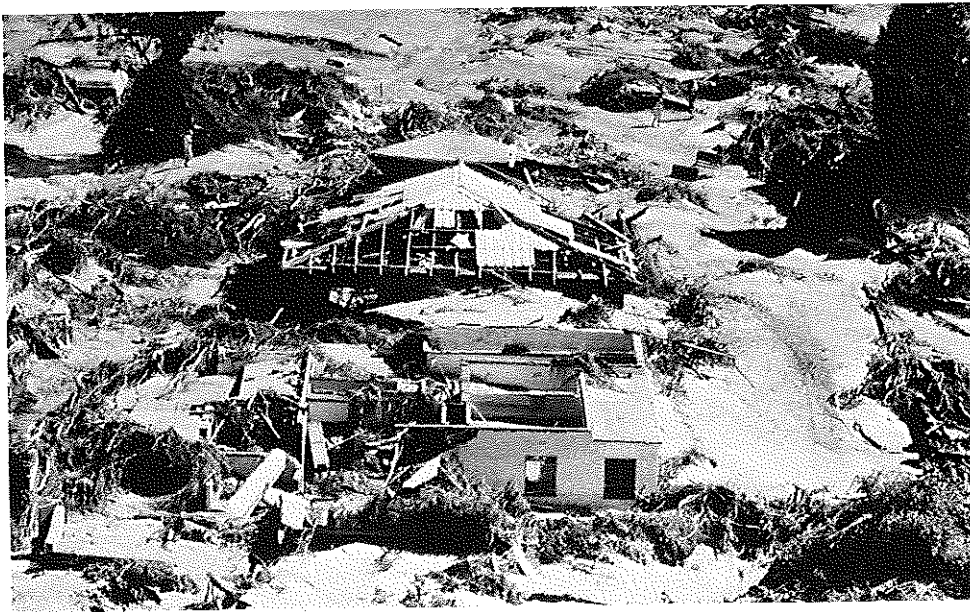
FIG. 11: Devastation of Laingsburg during the floods of January 1981 ( Die Burger , January 1981).
