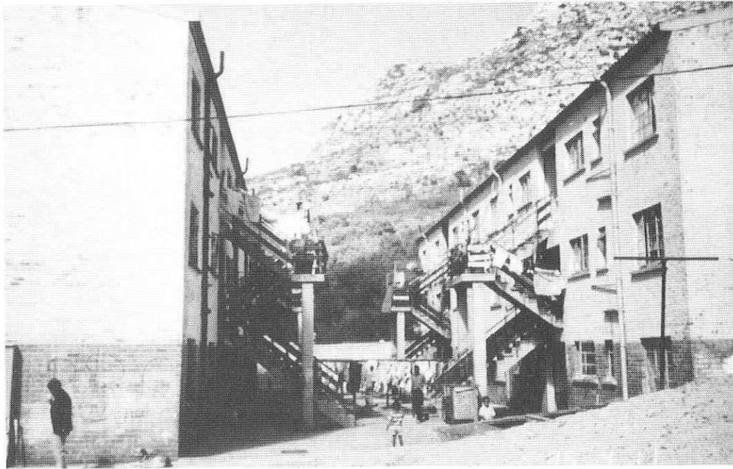
FIG. 23: High density, low-income apartments adjacent to the harbour area. (Photo: WCRSC).
