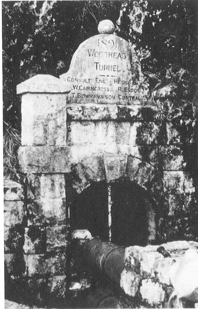
FIG. 9: In 1891 the Woodhead tunnel was completed; this 640m long tunnel led water from Disa stream through the mountain to Slangolie Ravine south of Camps Bay, providing Cape Town with a supply of potable water (Photo: Hout Bay Museum).
