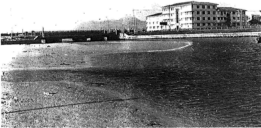
FIG. 17: Marine sand penetration upstream from the Royal Road bridge. Previously the water was ca 1,5 metres deep in the area now occupied by the sandbank.
