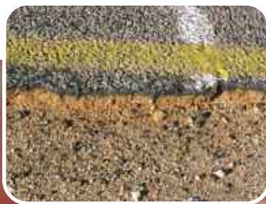
Left: A typical part of one of the marked sections of roads – see the hard self-stabilised lateritic base layer beneath the bitumen surfacing, which has given very good performance Below: A marginal quality silcrete used as surfacing aggregate in Botswana
