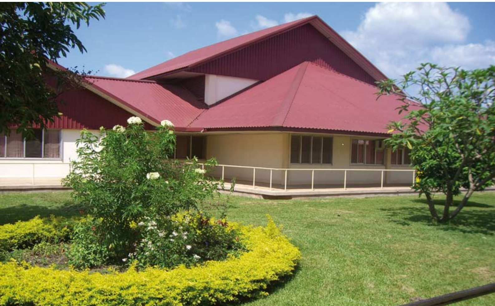
The 'shallow' plan of the building is responsive to the climate, using an open corridor system, which provides plenty of fresh air and light, and is separated by large, planted courtyards
