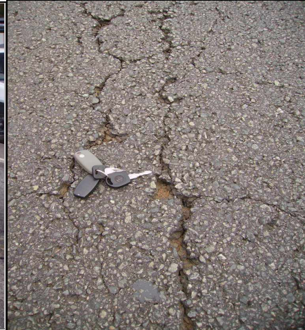
Figure 3: Cracked BRCA surfacing section P3
