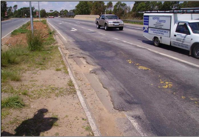
Figure 2: Permanent deformation at intersection road P2
