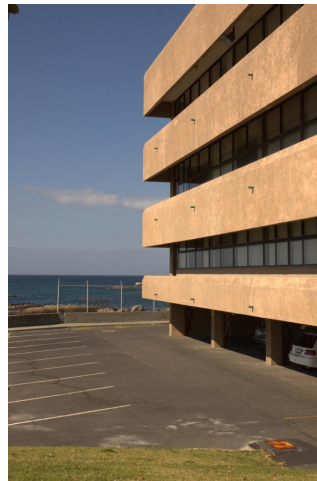
Figure 5: Balcony Parapets at IMT
